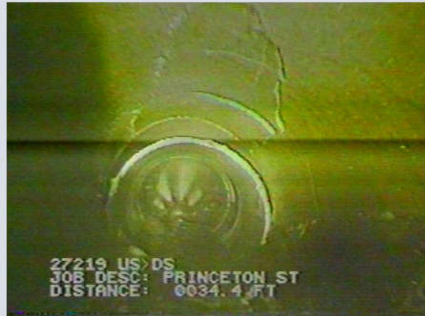
Displaced Joint
